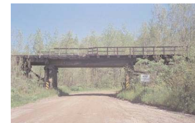
Skyline Parkway passes under this railroad bridge at Beck’s Road.
