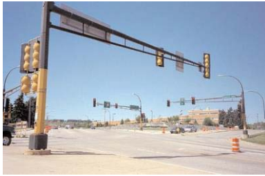
The Mesaba/Central Entrance intersection is difficult for pedestrians and bicyclists to navigate.
