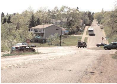
The Kenwood Avenue intersection is confusing and hazardous.
