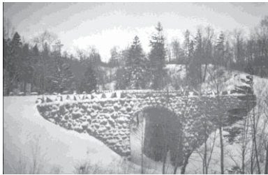
Stewart Creek Bridge in snow, date unknown. Source of photos this page: Northeast Minnesota History Center, UMD.
