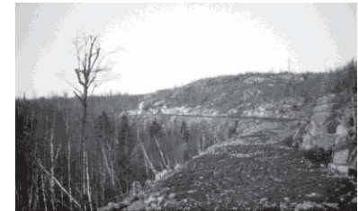
Bardon's Peak segment under construction in the 1920s. Photo: F. Rodney Paine.
