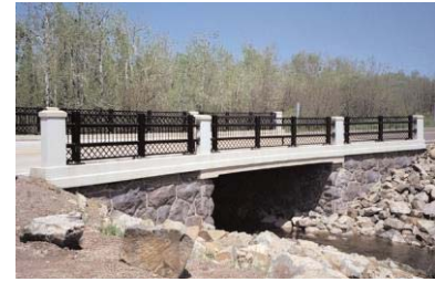
The new Keene Creek Bridge
