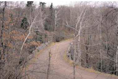
Stewart Creek bridge in late Fall.
