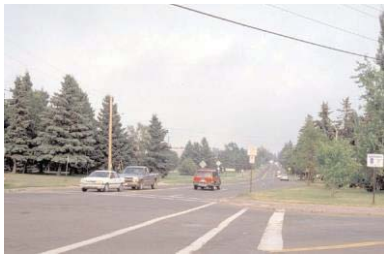
College Street and Junction Avenue, a confusing intersection for Parkway travelers.
