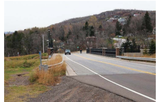
A motorist and bicycle crossing the new Skyline Parkway bridge over Piedmont Ave/Trinity Rd. (US 53.)
