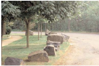
Native rocks are used as guard stones along the parkway.
