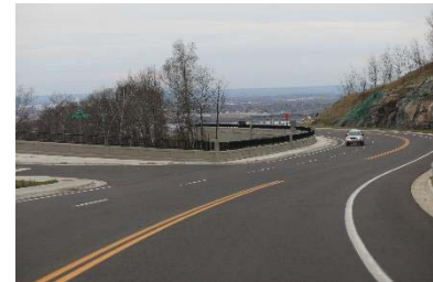
The reconstructed Haines Road intersection
