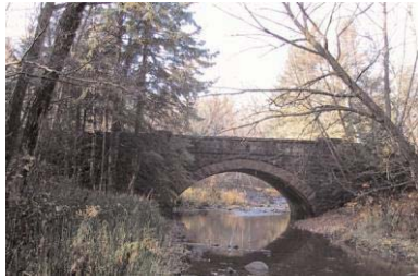
Historic bridge #4 on the Seven Bridges segment.
