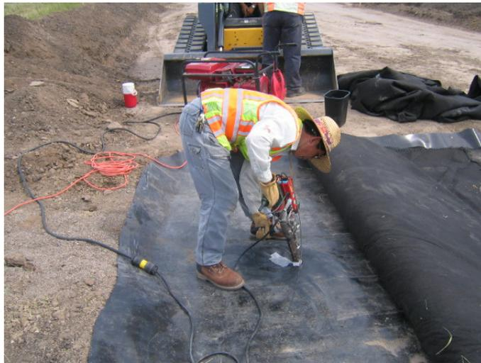
Figure 2. Installation of Lysimeter
