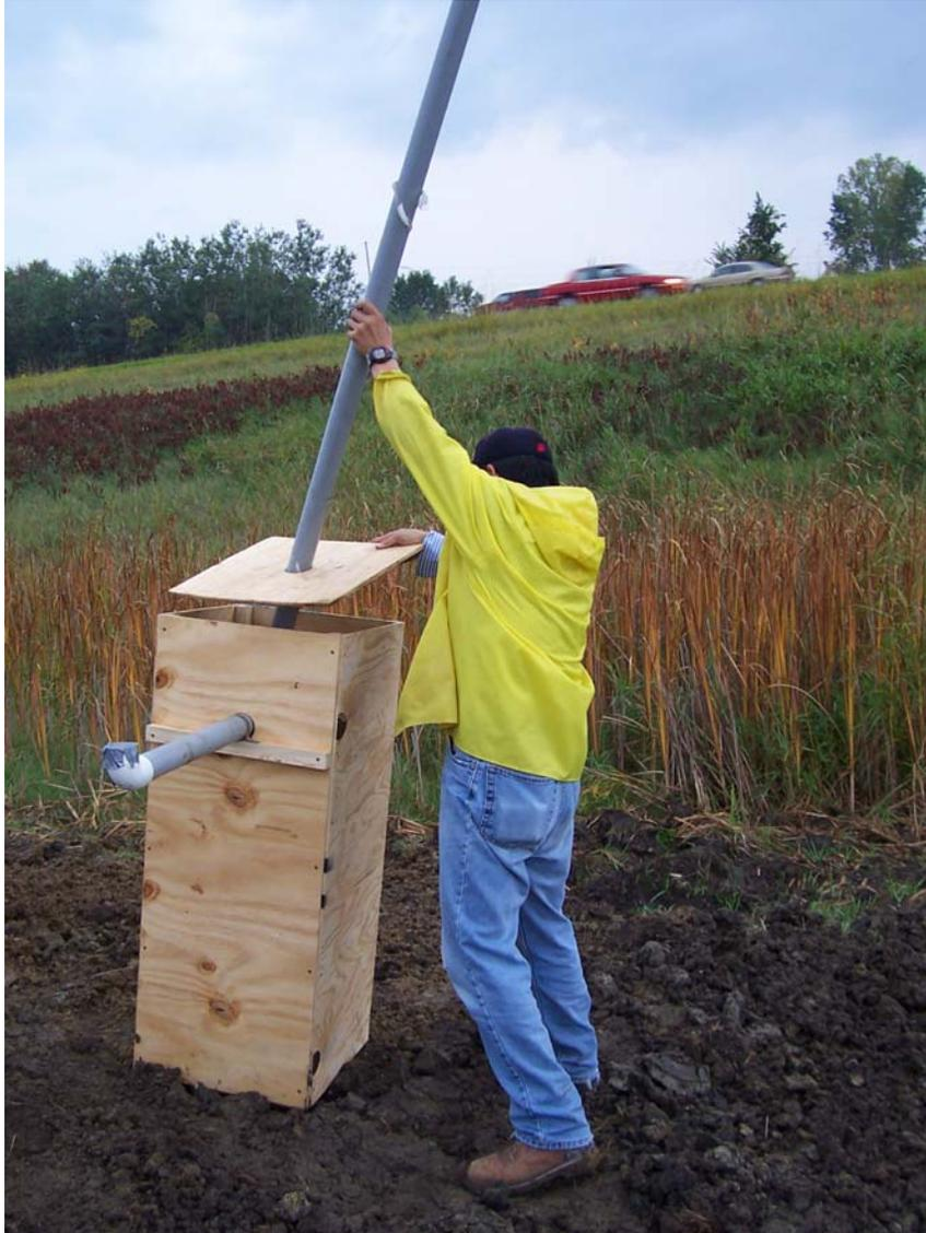
Fig. A-6. Assembling leachate collection tank.
