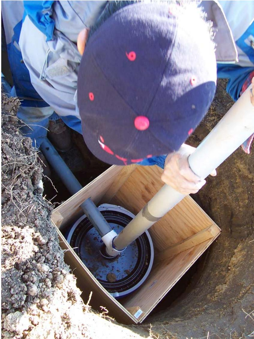
Fig. A-7. Installing leachate collection tank.
