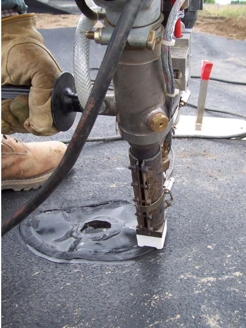
Fig. A-4. Welding geomembrane to lysimeter drainage pipe assembly.
