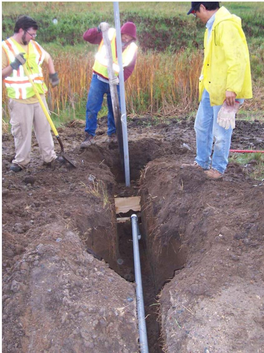
Fig. A-8. Installing leachate collection tank.
