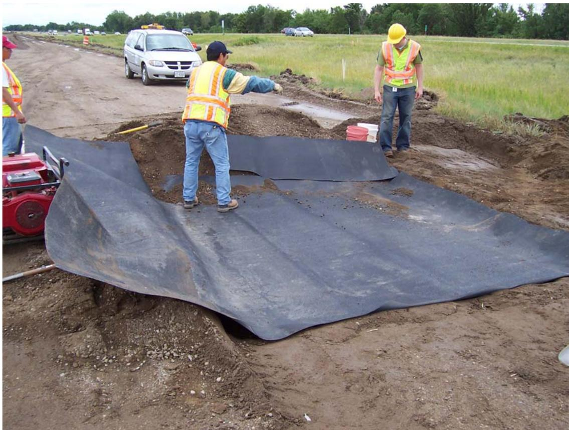
Fig. A-3. Installing geomembrane for lysimeter.
